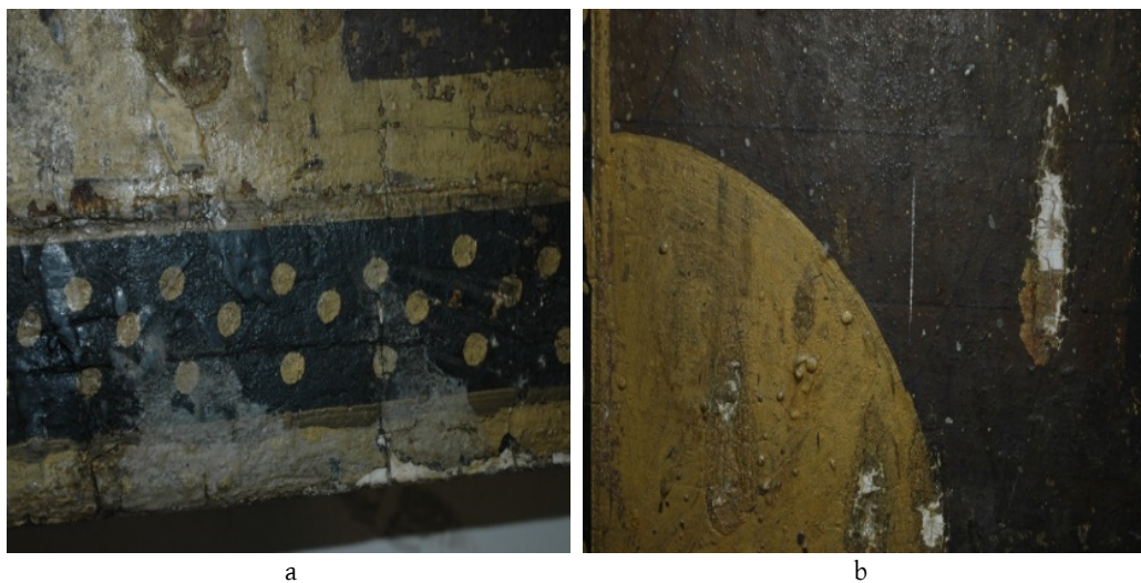
Figure 6. a – flaking of the preparation layer; b – wearing and fading of colours
