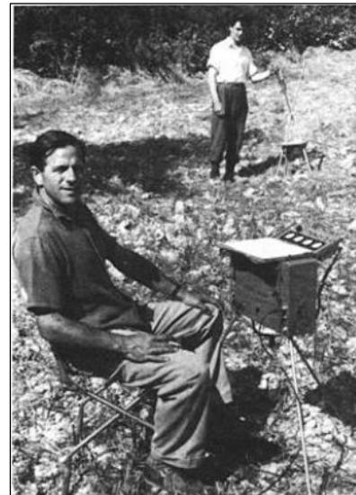
Figure 1. Martin Aitken using the prototype of the proton magnetometer (Clark, 1990)
